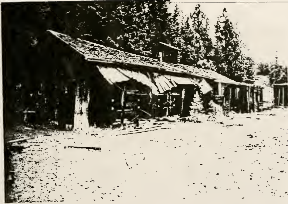
Figure 131. Blacksmith's Shop (structure #43), east view.
